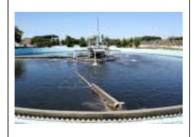
Jeju Western Wastewater Treatment Plant serves four districts including Aewol, Hallim, Hangyeong, and Oedo. With a treatment capacity of 24,000 m³ per day using the advanced SBR (Sequencing Batch Reactor) method, the facility plays a vital role in regional wastewater management. Equipped with extensive pumping stations, pipelines, and reuse facilities, it also supplies 5,000 m³ of treated water daily for agricultural use.
