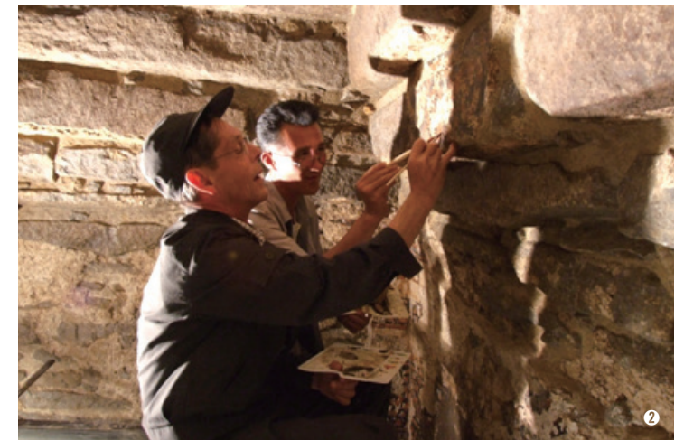
① Installation of protective glass walls for tomb murals in Yaksuri ② Preservation work on tomb murals in Susalli
