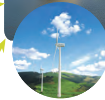
Wind power plant
