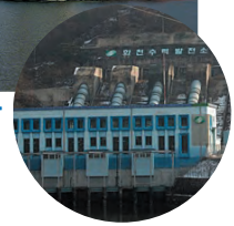
Hydroelectric power plant
